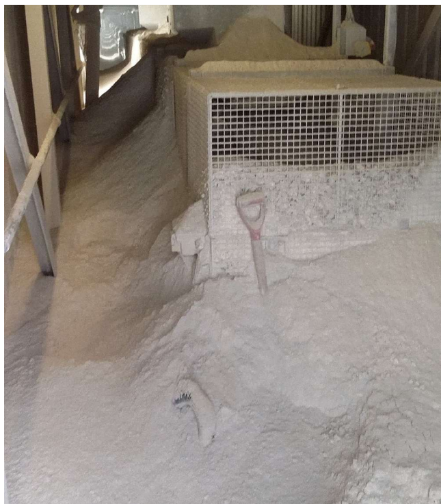
Piled high enough to encapsulate the tail pulley and belt, the dust was a serious problem.
